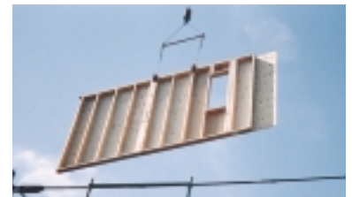
Lifting of wooden panels
