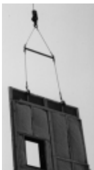
Lifting of wooden panel
