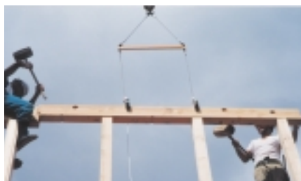
Lifting of wooden beam
